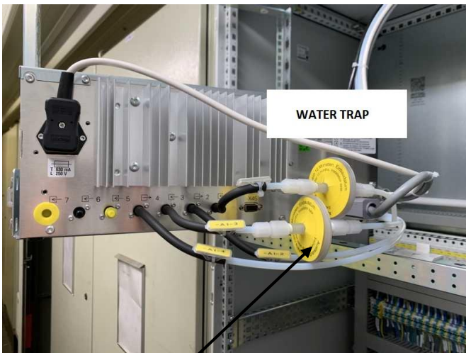
2 x Watertrap model 205N cConnected before analyzer (2 measuring channels)
